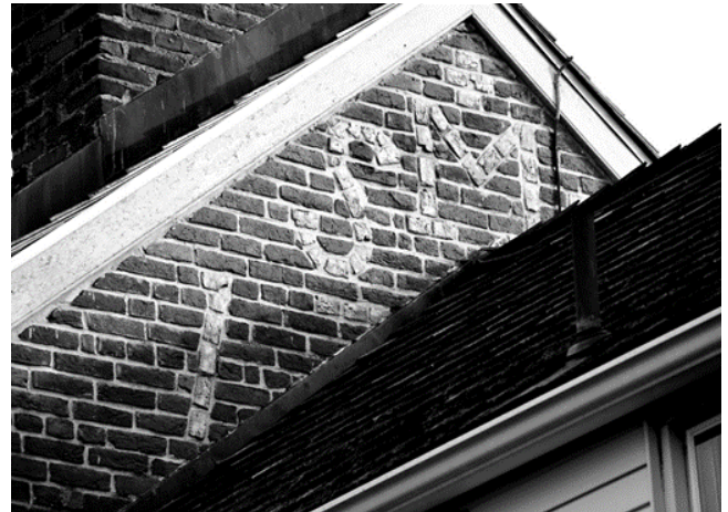
Figure 2. Mayhew house. View of the initials of Stanford and Esther Mayhew from the north side. The "1" and the top of the "7" of the year 1762 are visible. A 3-course diamond sits over the "M."
