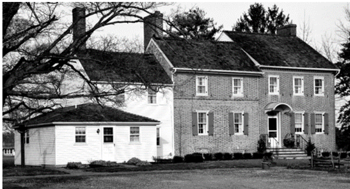
Figure 1. Mayhew house on Newkirk Station Rd, Upper Pittsgrove. The brick sections were built by Stanford and Esther Mayhew, 1762 (center) and Eleazar and Sarah Mayhew, 1792 (right). The center house originally had a central door and a pent roof over it. The opposite side was the front of that house. Before 1950 its roof was higher and totally covered the initials and date of the center section. John Seabrook purchased it and lowered the roof to reveal the initials of Stanford and Esther Mayhew and portions of the year 1762. 3 Photo ©2020 Janet L. Sheridan
