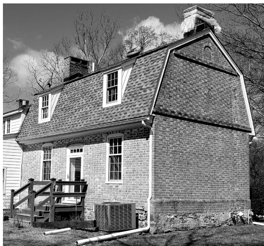
Figure 8. Jacob and Catherine Richman house, 1746, Upper Pittsgrove. Two facades are Flemish checker bond. Decorations include two Flemish checker string courses, checkered segmental window/door arches and a date plaque. Photo ©2020 Janet L. Sheridan
