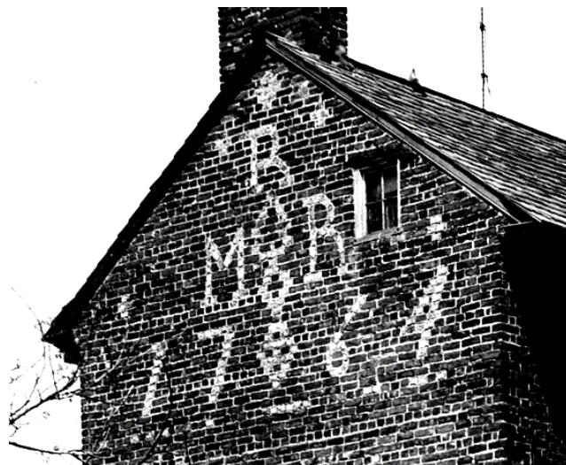
Figure 5. Michael and Rebecca Richman house, 1764, Upper Pittsgrove. The coronet is the uppermost shape below the upper "R." Photo from Historic American Building Survey HABS NJ,17-PIT. https://www.loc.gov/pictures/collection/hh/
