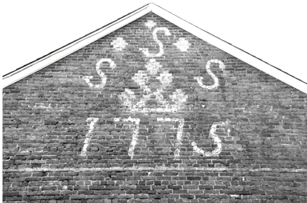
Figure 6. Samuel and Sarah Swing house, 1775, Upper Pittsgrove. These white bricks are rare. Photo ©2020 Janet L. Sheridan
