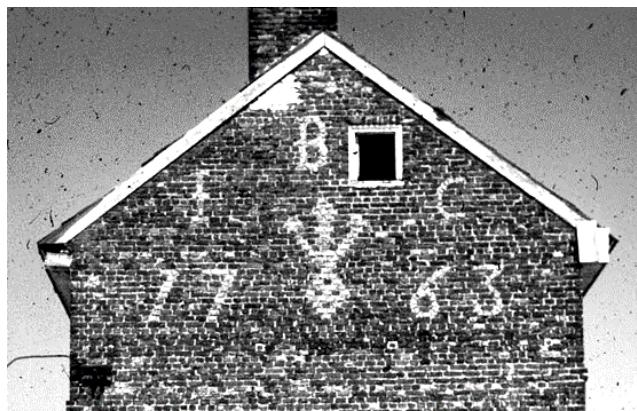
Figure 4. John and Catherine Biddle house, 1763, in Carney's Point (formerly Upper Penn's Neck), demolished 1980s. Photo by and courtesy of Dr. David Orr.
